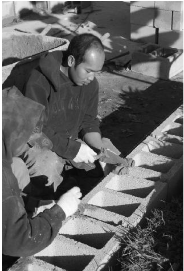
Brickmasons, blockmasons, and stonemasons usually work outdoors.
